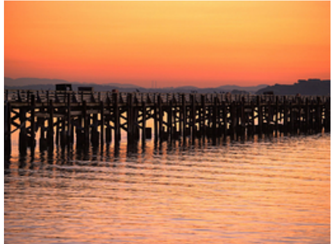
Ground zero for the Marin County desal plant
